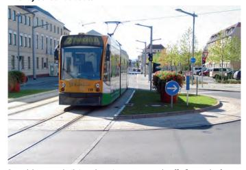
Roundabouts are built in order to improve general traffic flow and safety. For public transport they often have a negative impact by reducing travel speed and comfort for bus passengers and drivers. A public transport priority solution for roundabouts would have special traffic signals for tram or bus running directly through the middle of the roundabout. Example from Nordhausen, Germany. PHOTO: GUSTAV NIELSEN
